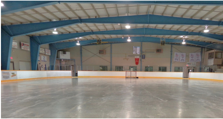
Before the install
