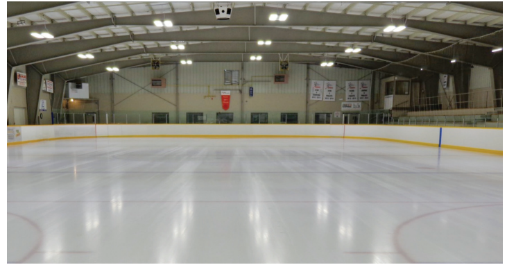
After the install
